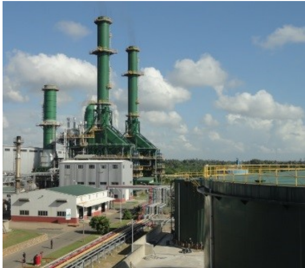
Figure 1: General view of the Yugadanavi 300 MW CCPP
